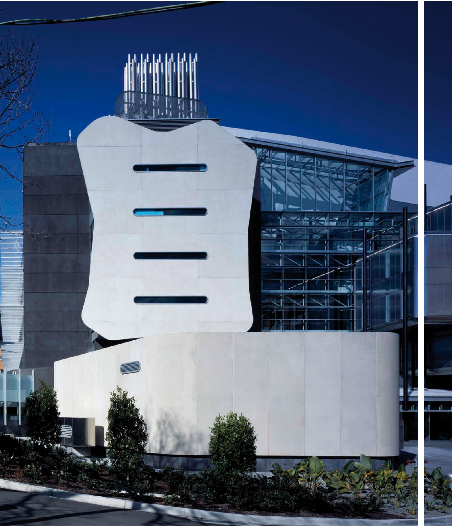
The David Pennington Bio 21 Institute Building, University of Melbourne, designed by DesignInc Melbourne Photographer Trevor Mein
